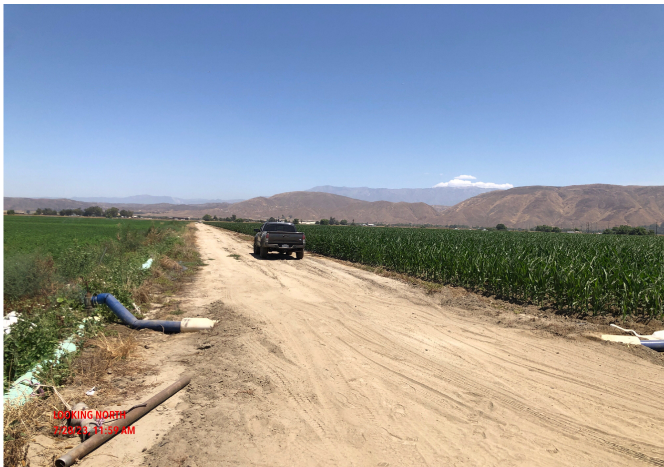
Photo 18 Irrigation water delivery system
